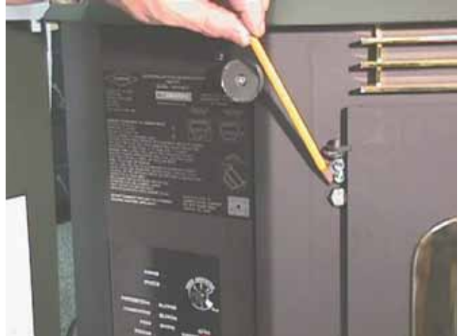
Fig.15: Draft Meter bolt hole location
